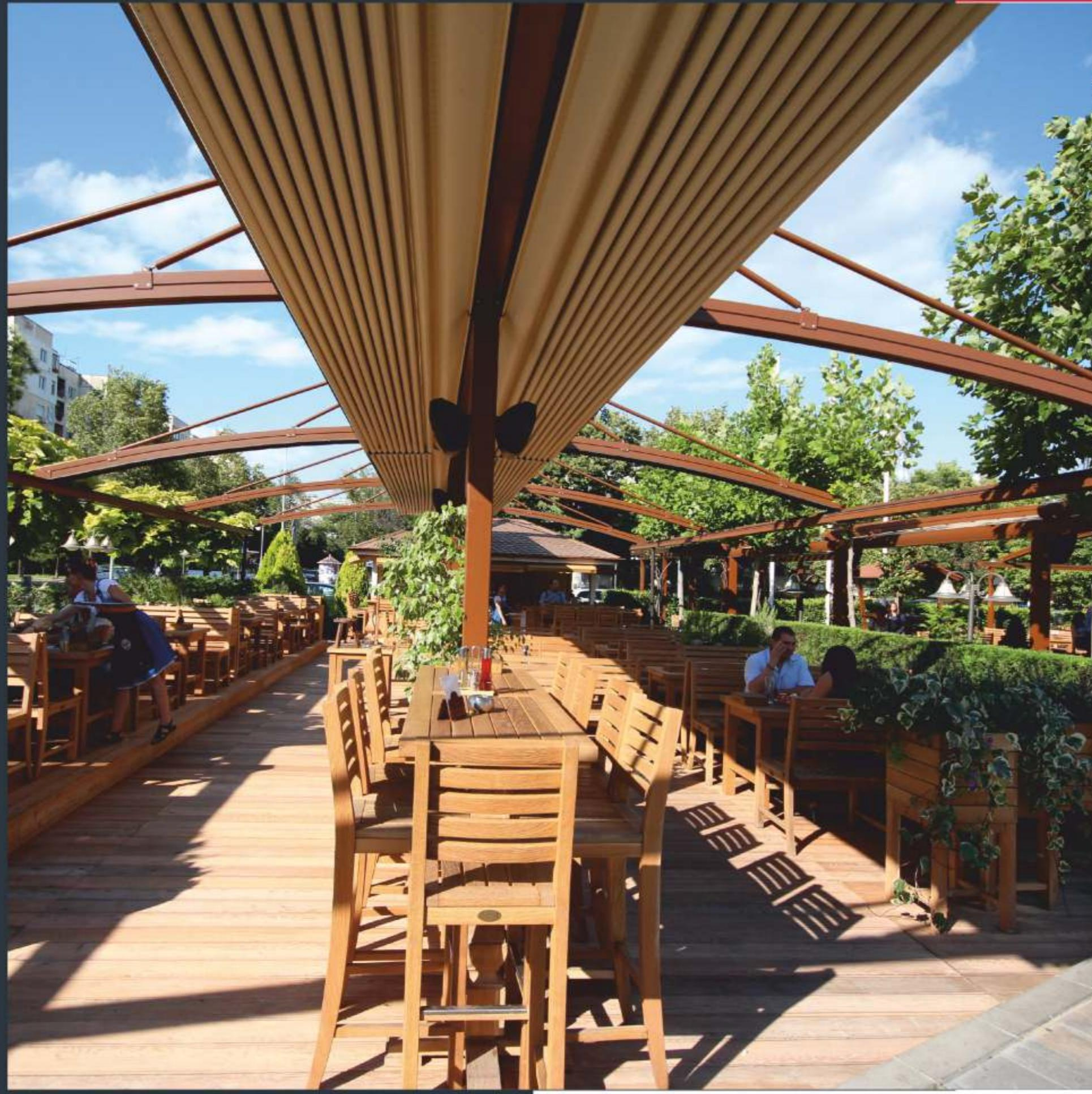
The SPLINE VARIANCE Curved Rafter Profiles have been designed with smart side channels that allow an easy installation and side Waterguard Channels. Rafter profiles, including a timing belt of T10/33, are driven by patented six-wheel sliders with easy clip installation for fabric that allows a silent motion when the fabric is retracted. SPLINE VARIANCE rafters are served with two different dimensions:
